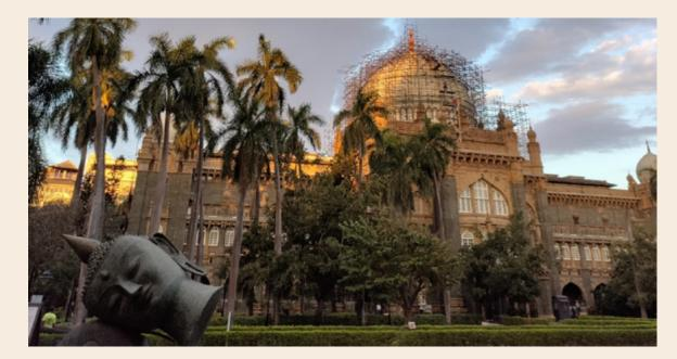
a very long duration, which otherwise, during a normal working of the museum, would have been impossible. The structural study of the dome revealed that the repairs done in the 1970s by guniting have prolonged the life of the dome. Its waterproofing done with China mosaic was found to be efficient and was repaired locally as required after monitoring it for two years.
