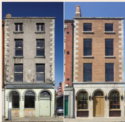
➤ 18 ORMOND QUAY BEFORE (2016) AND AFTER (2020)
